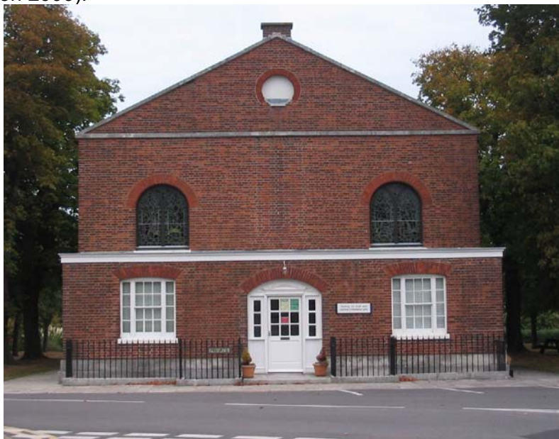
Figure 8: South-West elevation - photograph
