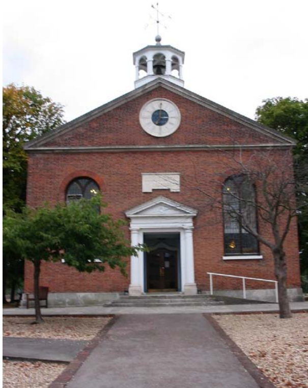
Figure 5: North-East elevation - photograph
