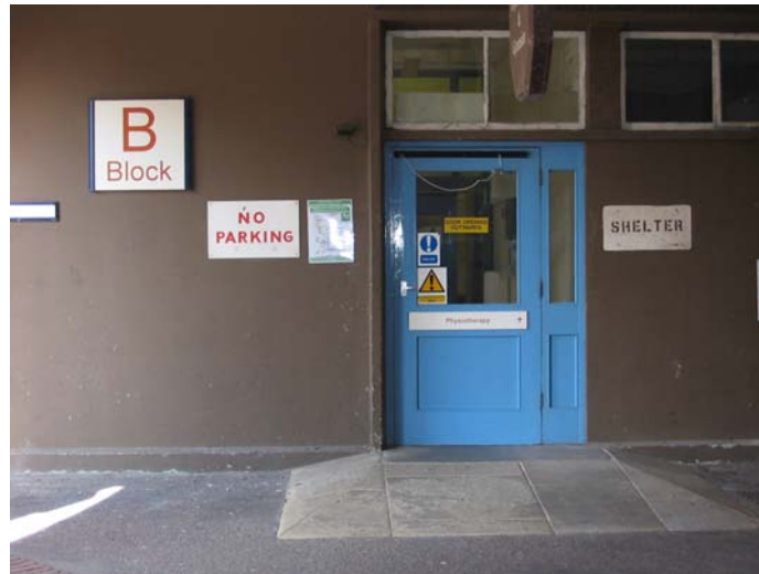
Figure 6.5: Shelter sign B Block
