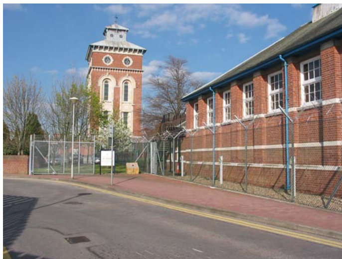
Figure 7.3: Modern security gates and fencing
