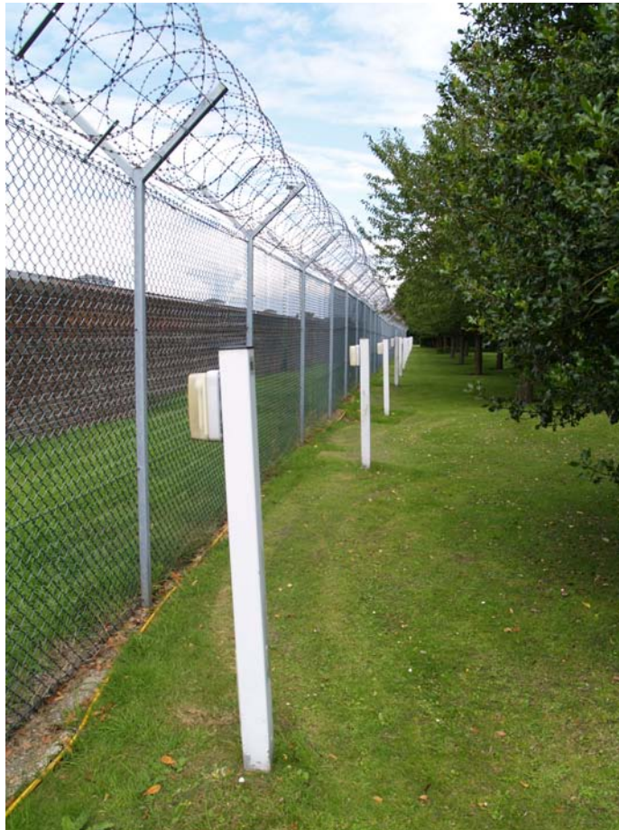
Figure 7.2: Modern security fencing and lighting
