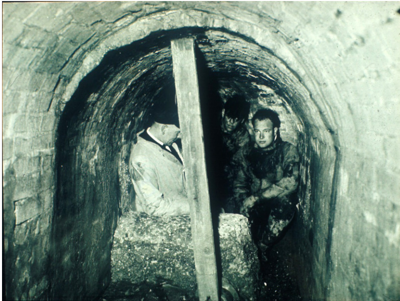
Figure 5.15: Main Hospital Sewer
