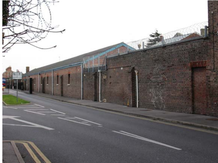
Figure 5.25: North East Perimeter wall looking south
