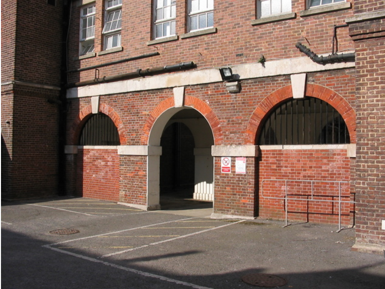
Figure 5.10: Extant wall and grill 'F' Block
